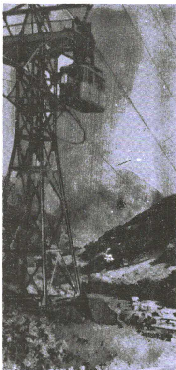
Galzig-kabelspoor St Anton am Arlberg
